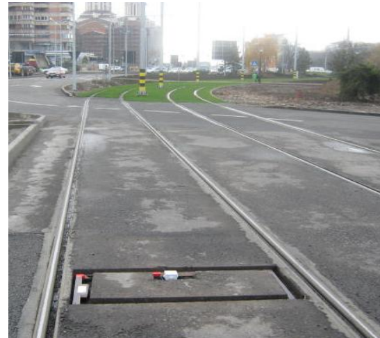
Fig. 7. - Detail location,, inductive loop closure "for the detection tram in the asphalt [1]
