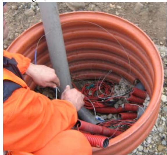
Fig.8.- Fireplace input protection tubes stranded copper conductor, which is connected with the automatic traffic light [1]
