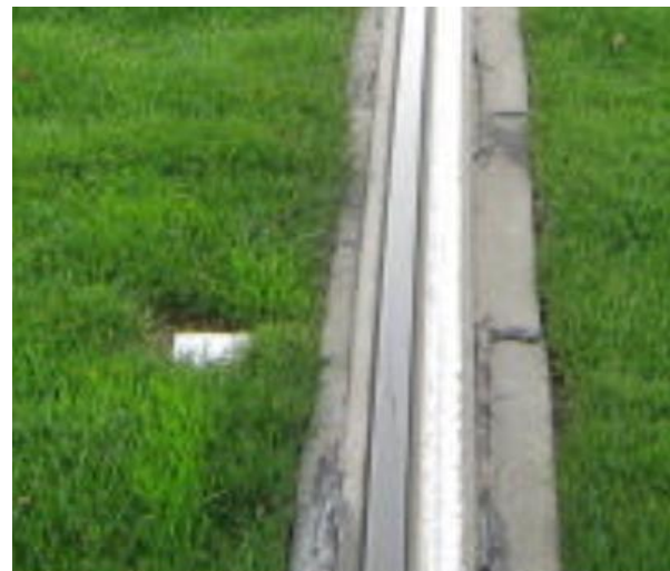
Fig. 4. - Covering natural grass inductive loop detection tram grassy area [1]
