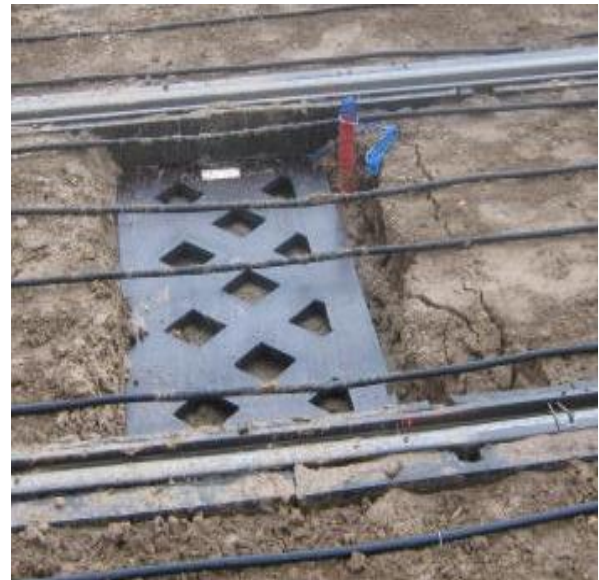
Fig. 3. - Detail Location inductive loop detection anticipation tram grassy area [1]
