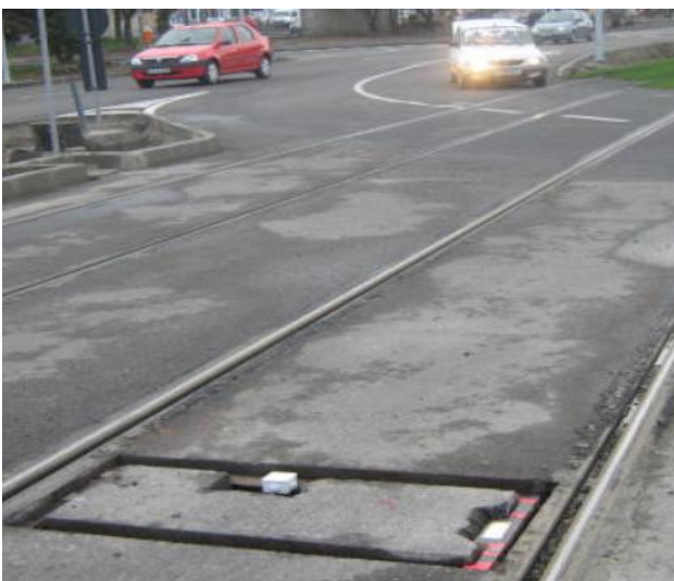
Fig. 6. - Detail Location inductive loop,, safety "for the detection tram in the asphalt [1]
